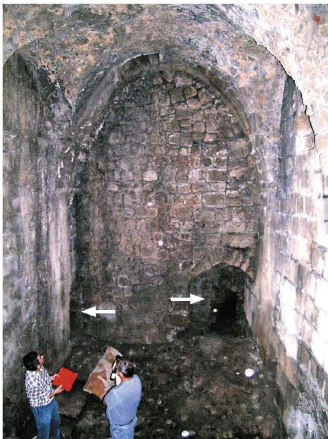
*Fig. 27.1. Cistern 9, looking west; note the stairs on left and the tunnel to Cistern 9a on right (arrows).*
