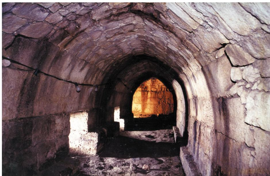
Fig. 27.10. *The Latrine Complex: Main Sewage Tunnel, looking north; note the vaulted ceiling and the openings of the two eastern connecting tunnels into the Latrine Complex at left.*
