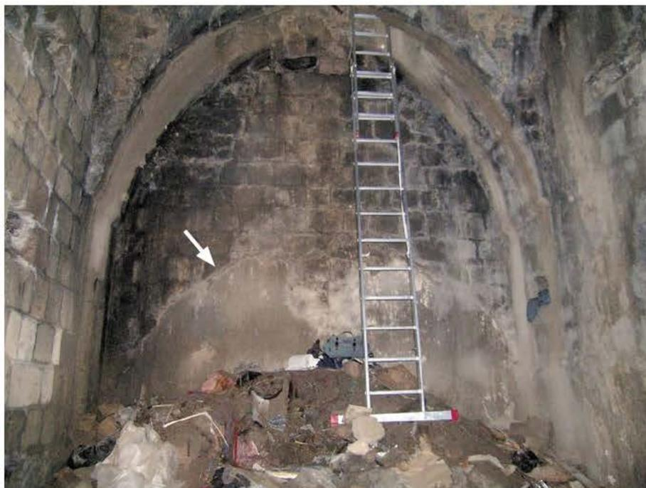
*Fig. 27.2. Cistern 9, looking east; arrow marks the line of plaster of the early stage of cistern construction.*
