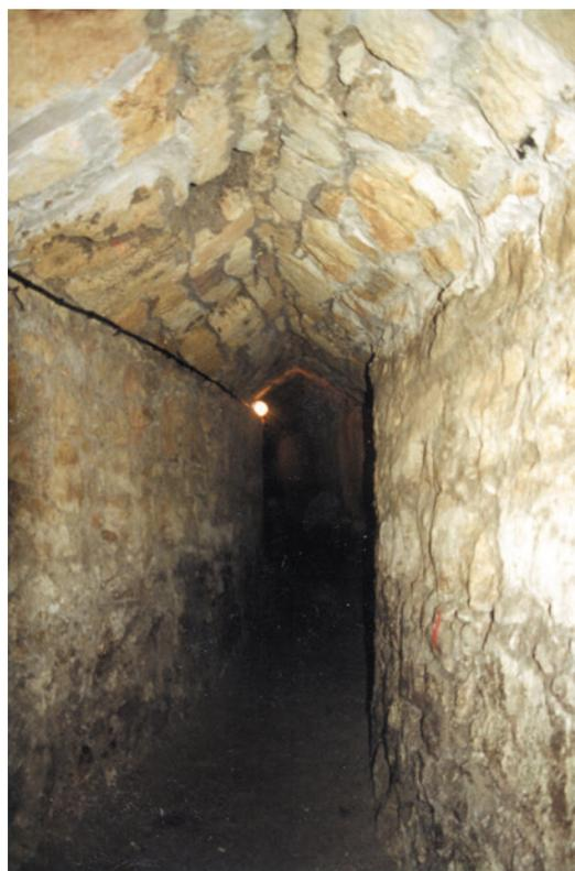
Fig. 27.11. *The Main Sewage Tunnel of the Hospitaller Compound; note the gabled ceiling.*
